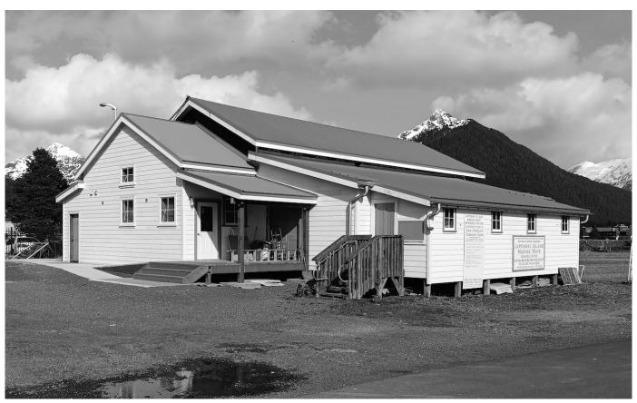
Northwest view, Japonski Island Boathouse (2024) - looking Southeast (no siding under upper gable eaves, no handrails, uneven ground)
