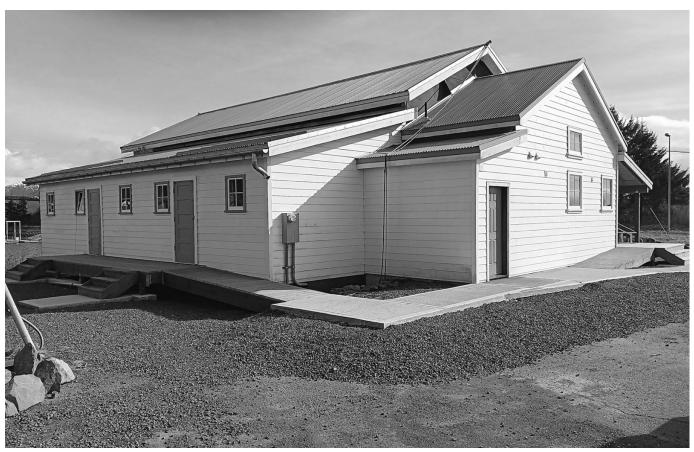
Northeast view, Japonski Island Boathouse (2024) - looking Southwest (no handrails on decks or ramps & several inch height discrepancy between concrete pads and surrounding yard)
